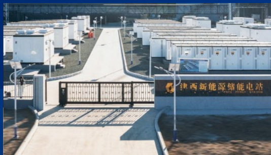
Jinxi New Energy User-side 60MW/120MWh Energy Storage Project
