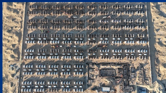
Inner Mongolia Dengkou 500MW/2000MWh Energy Storage Project
