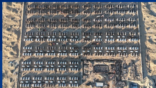
Inner Mongolia Dengkou 500MW/2000MWh Energy Storage Project
